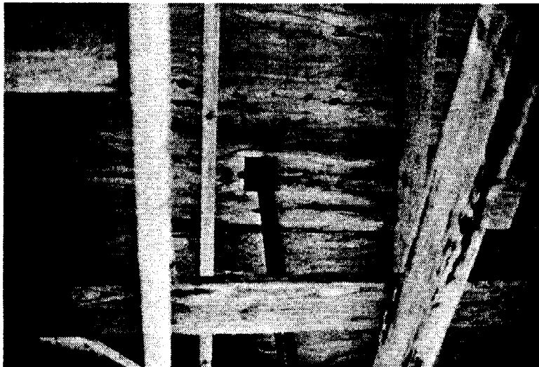
Figure 8. Plywood Sheeted Roofs
