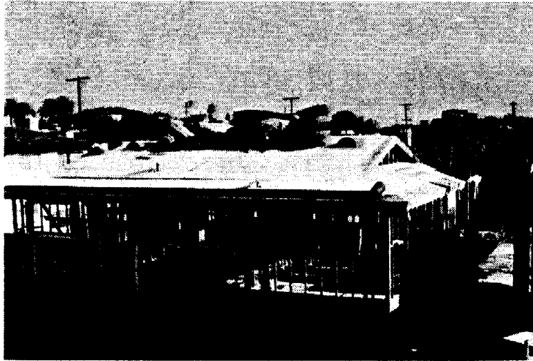
Figure 9. Treatment with 90 lb Roofing Paper.
