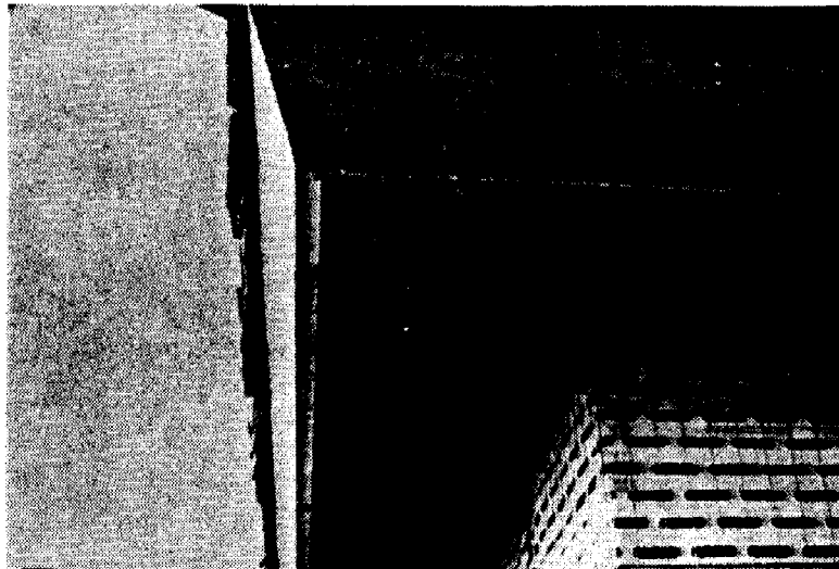
Figure 10. Wire Mesh Supports for Exterior Plaster is Carried under Eaves
